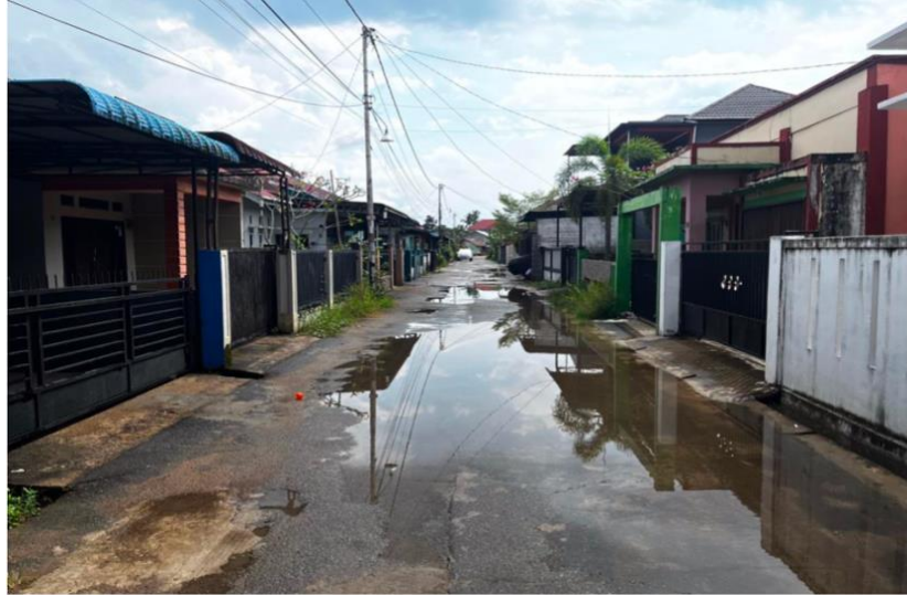
Figure 1. Existing Conditions of the Drainage System
