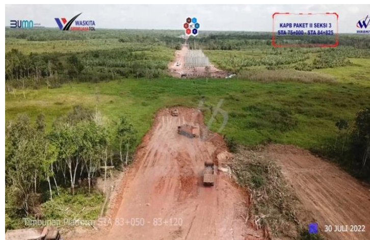
Figure 2. Embankment placement for platform construction before pile foundation installation.
