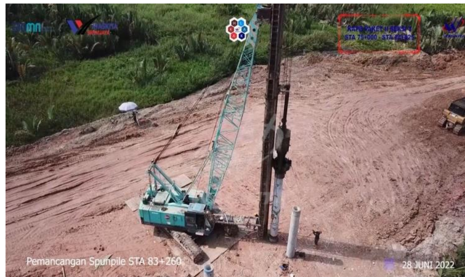
Figure 3. Pile Foundation Installation in Progress Using Platform Method
