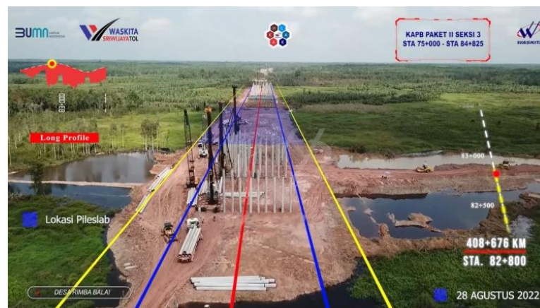
Figure 1. Swamp area at STA. 82+800 of the Kayu Agung–Palembang–Betung Toll Road Phase II, Section 3.
